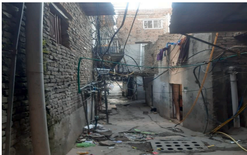
Fig. 6. Dangerous and Open Electric Connections (Source: Picture by authors).
