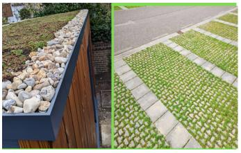
Figure X. Green Roof and water-retained pavement
