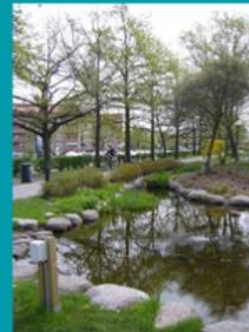
Drainage channel with vegetation filter
