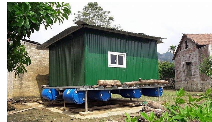
Adaptation Action: n. of houses made resilient to floods
