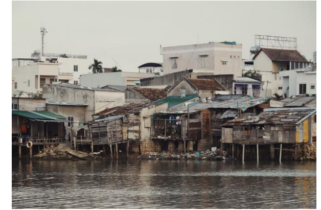
Vulnerable sector (building)
