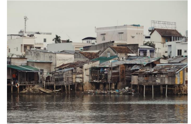
Vulnerable sector (building)
