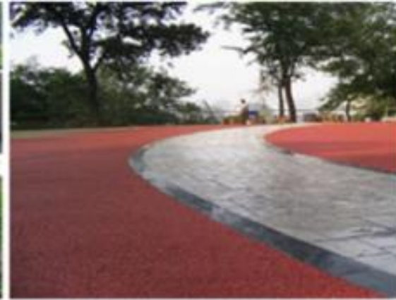
Permeable pavement
