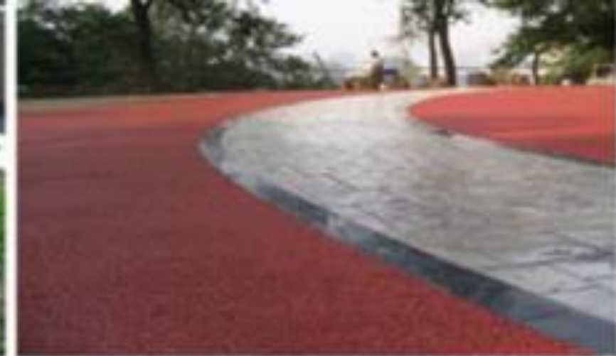
Permeable pavement
