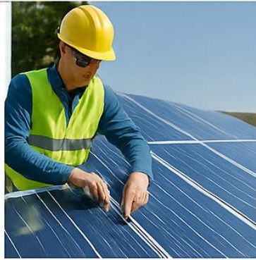
Resource Efficient Facilities
