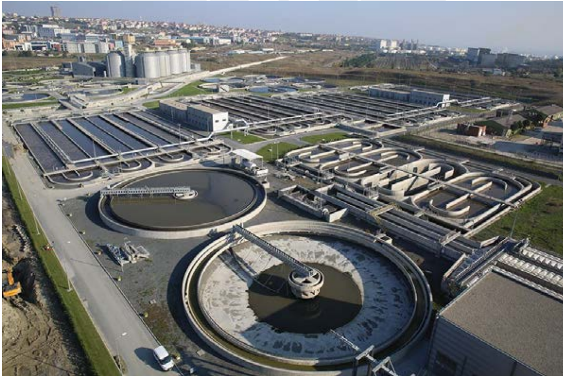
Ambarlı Advanced Biological Wastewater Treatment Plant
