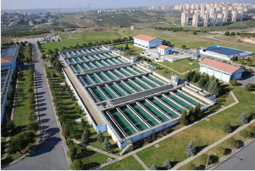
İkitelli Water Treatment Plant
