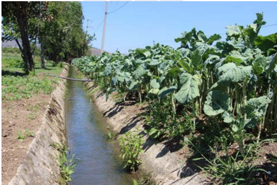
Irrigation Work with Open Concrete Channel System
