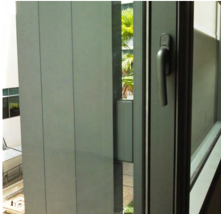
Figure 4.5.7: Double glazed operable window
