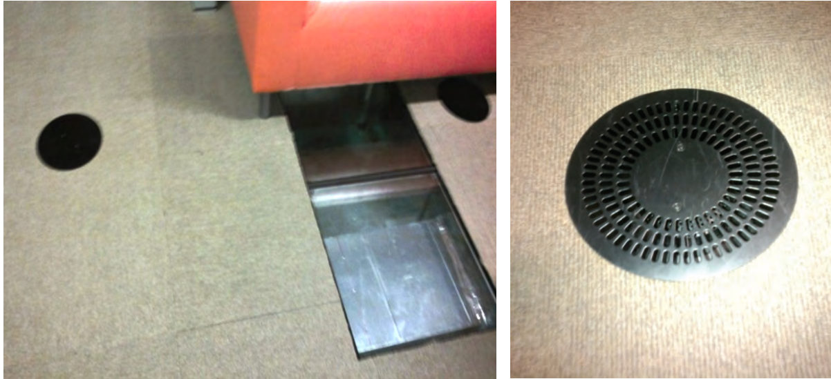
Figure 4.7.3: Displacement ventilation
