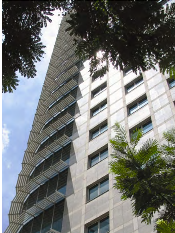
Figure 4.5.10: Low ETTV building façade made possible with appropriate wall to window ratio, sufficient sun shading devices among other technologies for buildings in the tropics
