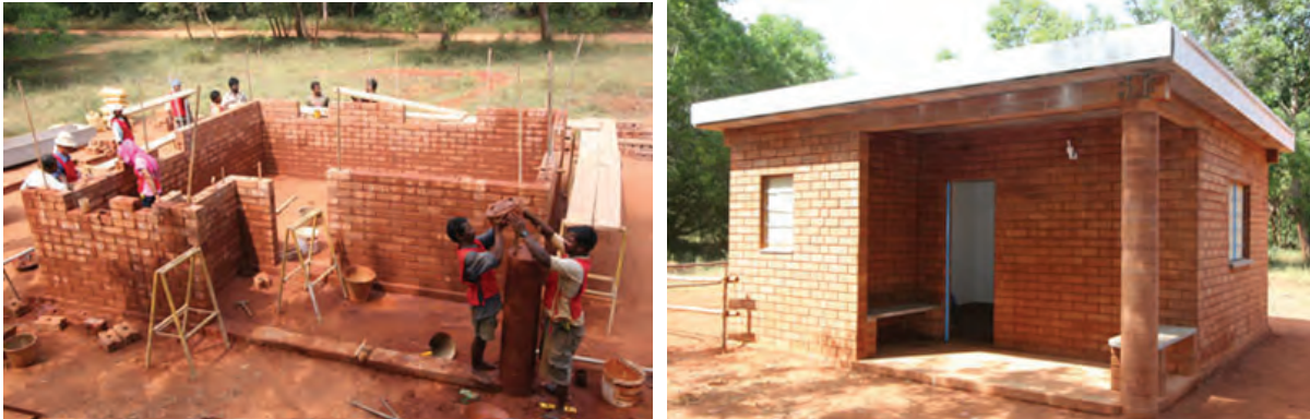
Figure 4.1.5: Movable house in Auroville, India under construction (left) and completion (right)
