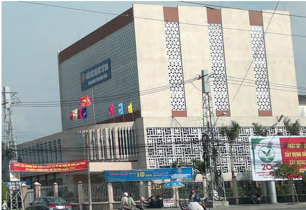
Figure 4.5.9: Solid wall application in combination with natural ventilation and daylight penetration for a bank in Vinh Long City, Vietnam
