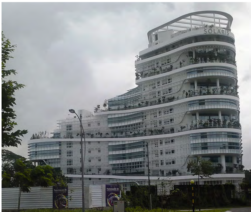
Figure 4.11.8: An effort to promote urban biodiversity by providing planting strips, connecting greenery on the ground to rooftop garden in the Solaris, One North, Singapore
