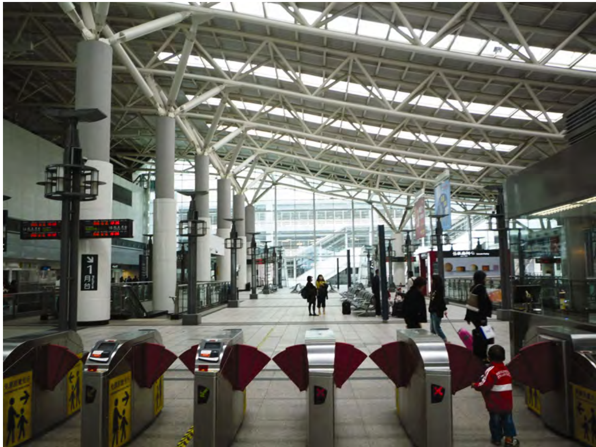
Figure 4.6.2: Reflective interior finishes enhancing day lighting performance in Zuoying Station, Kaohsiung City, Taiwan
