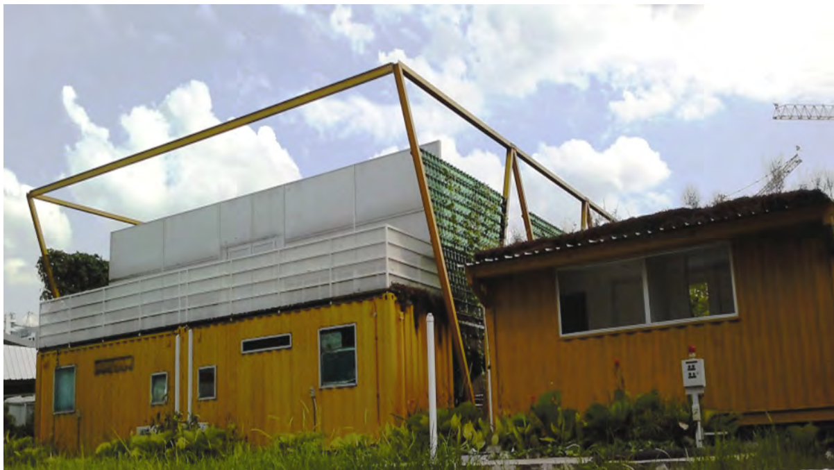
Figure 4.10.2: Shipping containers can be adaptively re-used in new buildings
