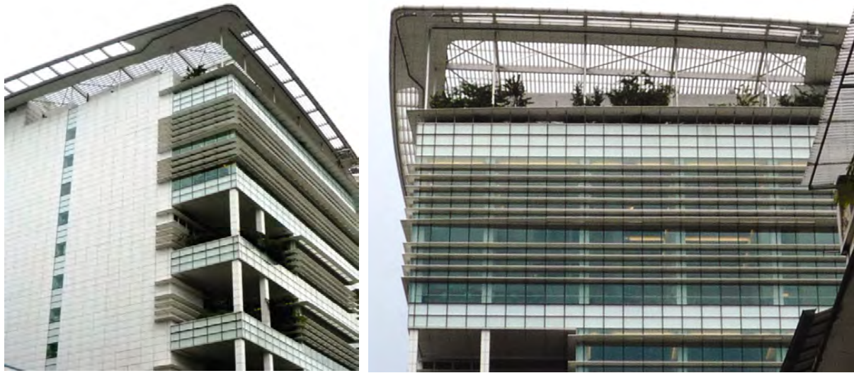
Figure 4.5.12: Low ETTV façade of the National Library Building in Singapore is made possible with double glazing, appropriate wall to window ratio and sufficient sun shading devices
