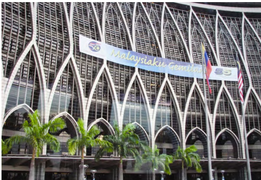
Figure 4.5.6: Sun shading devices integrated with traditional motif as architectural design expression for the Malaysian Ministry of Finance building in Putrajaya, Malaysia
