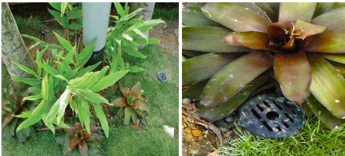
Figure 4.9.6: A drip irrigation system
