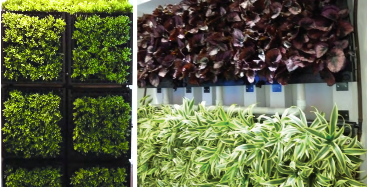
Figure 4.11.3: Green façade modular system embedded with irrigation and self drainage technologies
