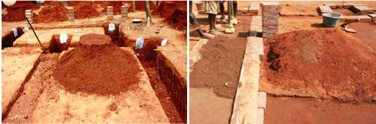
Figure 4.1.1: Stabilised rammed earth foundations under construction process in India
