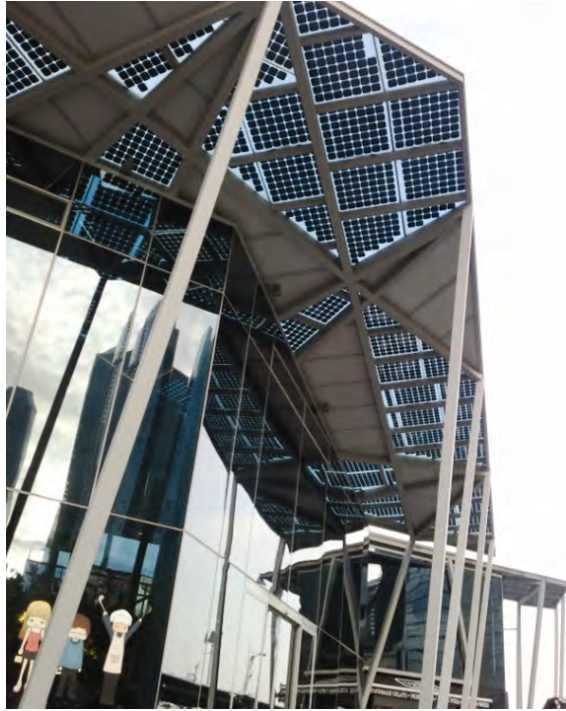
Figure 4.12.2: PV panels as integral part of building design
