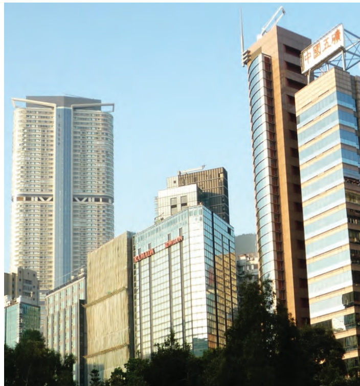
Figure 4.5.2: Wide range of building façades often found in urban fabric, such as Hong Kong in this illustration
