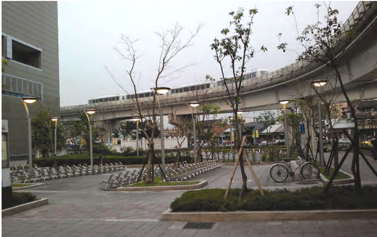
Figure 4.17.1: Sustainable transportation facilities in Nankang, Taiwan
