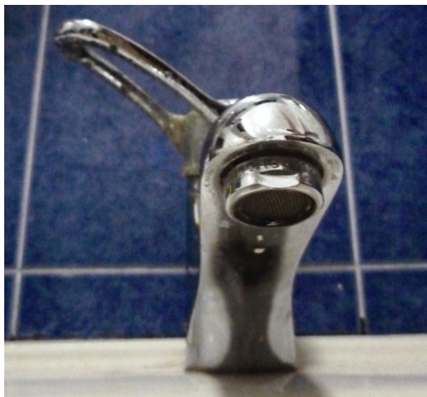
Figure 4.9.8: Aerator fixed onto a tap as a simple way to achieve water efficiency
