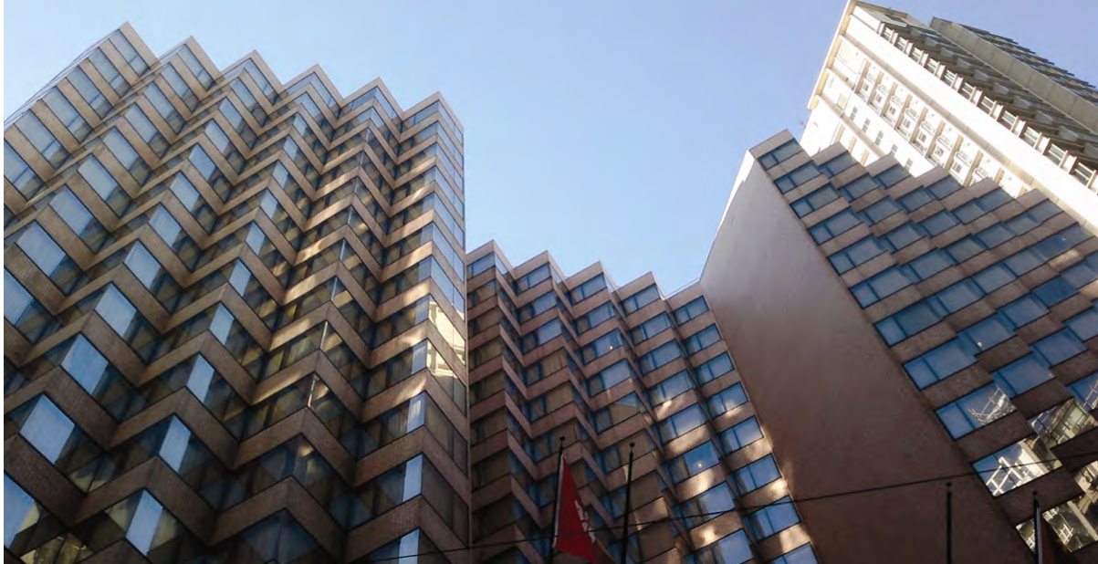
Figure 3.2.4: Building massing creates self-shading effect – i.e., most windows are shaded from the hot sunlight shining from the left
