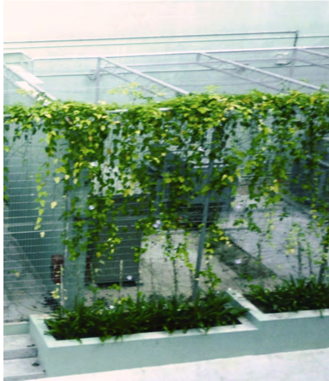
Figure 4.11.5: Support system green façade to cover a mechanical plant room
