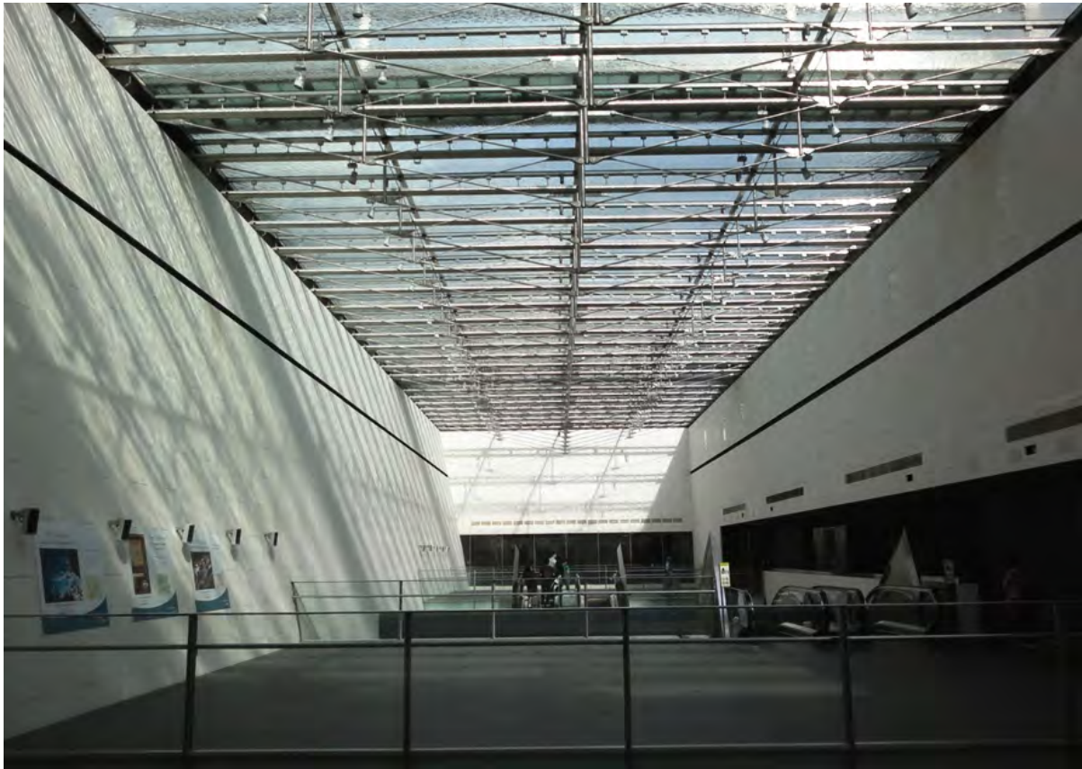
Figure 4.1.2: Modern application of water-roof system to bring benefits to both thermal comfort and daylight to building interior
