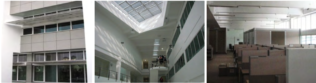
Figure 4.6.5: Light shelf, skylight and light pipe in Pusat Tenaga Malaysia’s zero energy office
