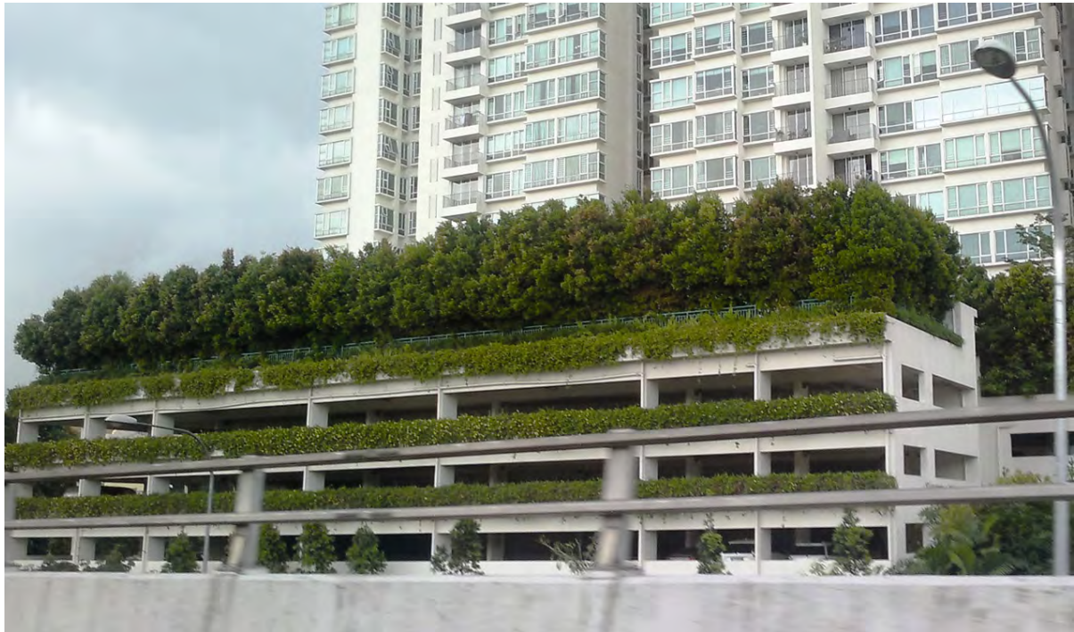
Figure 4.11.9: Green wall and roof greenery as environmental buffer for a residential development fronting a busy road
