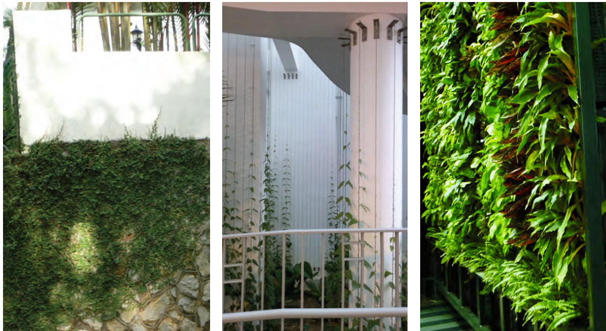
Creepers on wall surfaces
