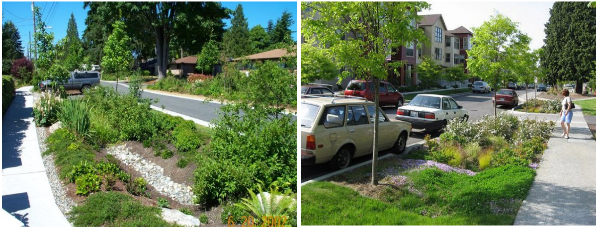
Figure 10: Example of a Rain Ditch in Seattle, US (EPA, 2017)
