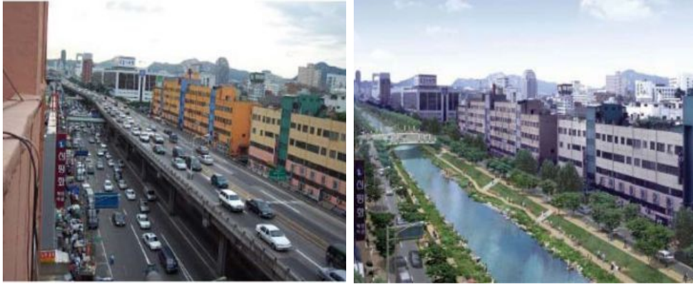
Figure 14: CheongGye River Before and After Ecological Restoration (Lee2006)
