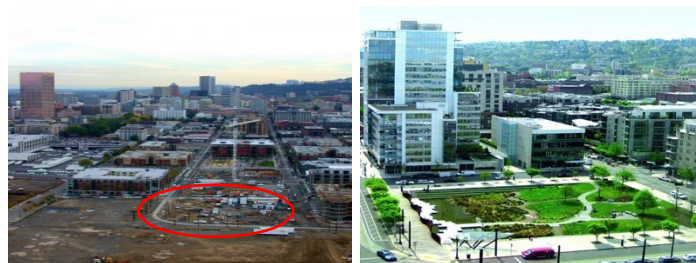
Figure 15: Tanner Spring Park Before and After Ecological Restoration 10
