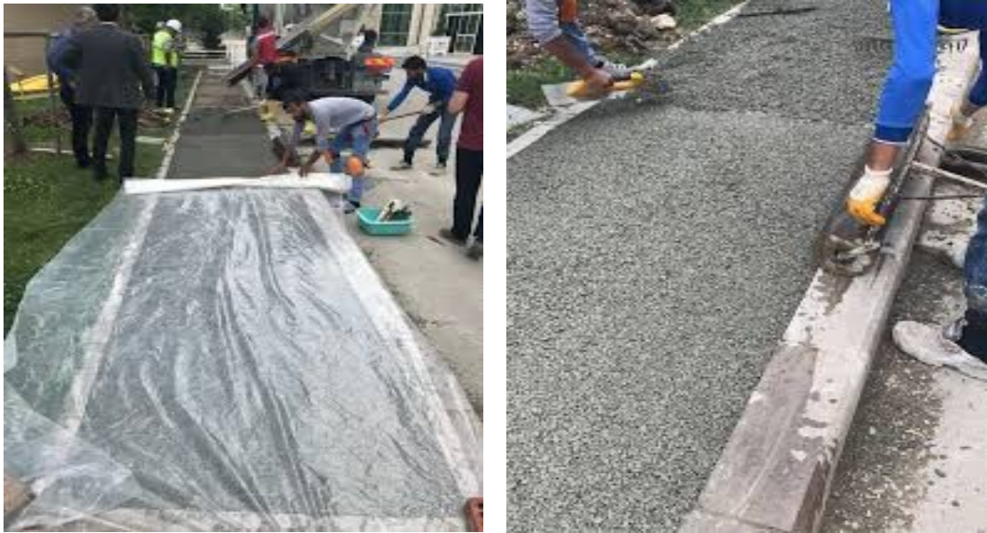
Figure 17: Ministry of Environment and Urbanization Permeable Concrete Application 12
