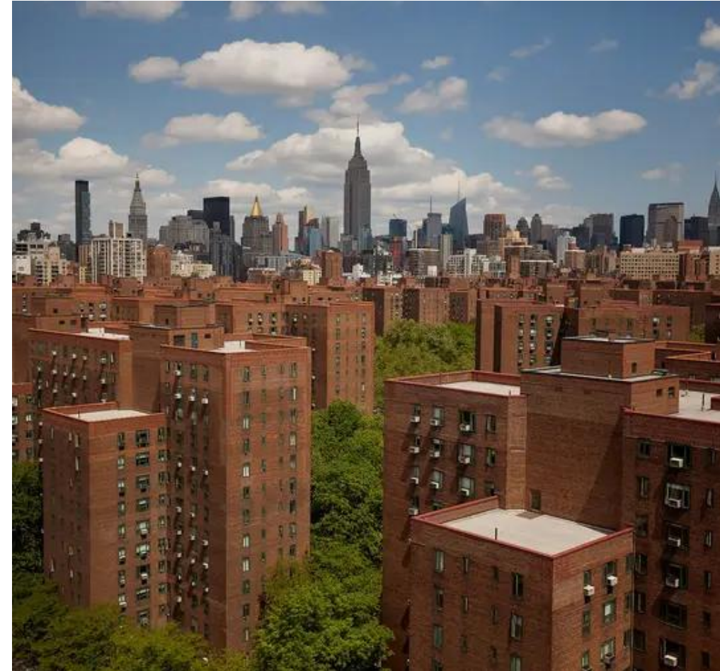
Stuyvesant Town–Peter Cooper Village New York City's residential building stock
