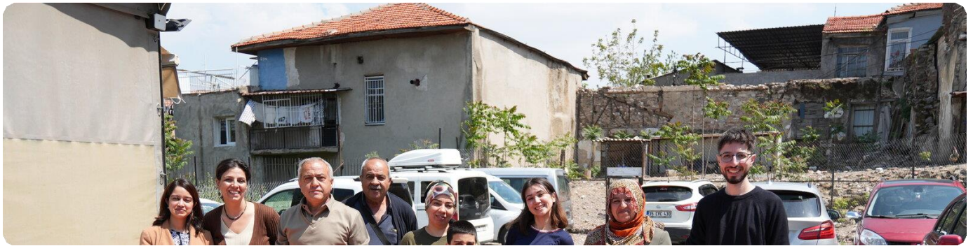
Modular flood barriers installed together with residents in Pazaryeri.
